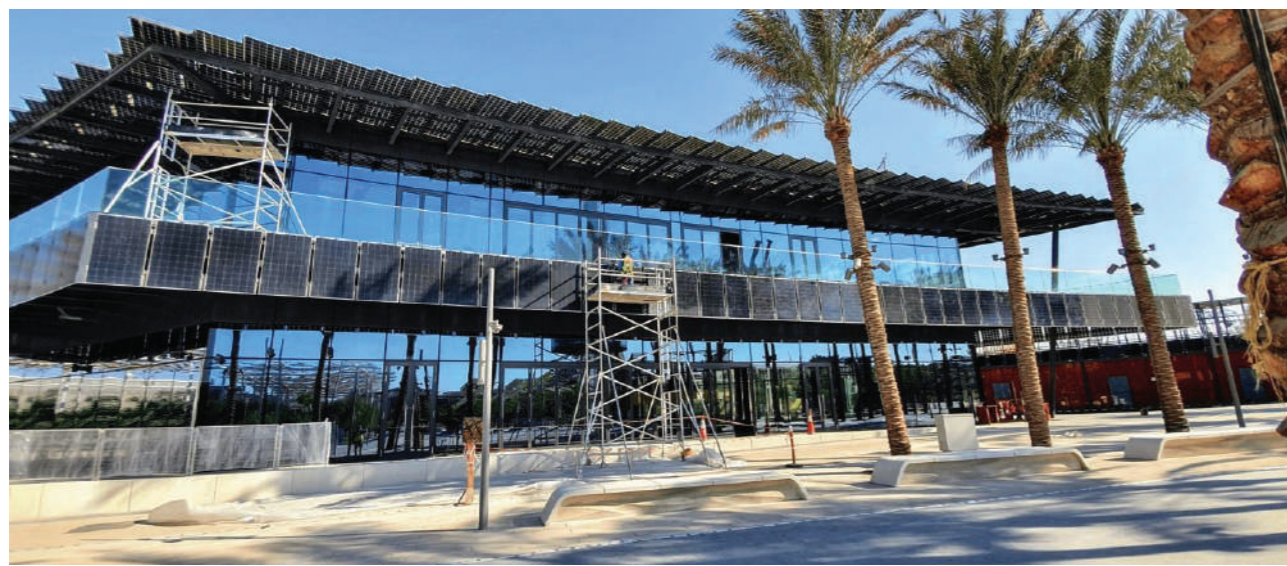
Figure (3): Restaurant Complex BIPV Integration in Canopies, Facades and Balustrades – Source: Empereal
